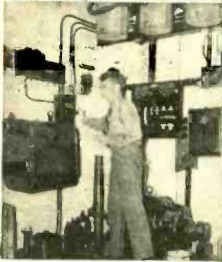
Lower left.—Starting the motor generators, high-voltage transformers and rectifying equipment needed to operate the huge Cyclotron. Upper left.—A luminescent beam of deuterons, made visible by the ionization of the air in their path. Top.—Watching the operation of the Cyclotron from a safe distance, in the control room at the University of Rochester. Upper right.—A nuclear physicist adjusting the gate leading to the bombardment chamber. Arrow points to the window through which the deuterons emerge. Bottom Right.—Starting the pump that evacuates the acceleration chamber.
